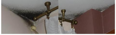
Fig. 5. Mold-covered upper wall corner below the balcony and ceiling comprising an extension of the balcony
